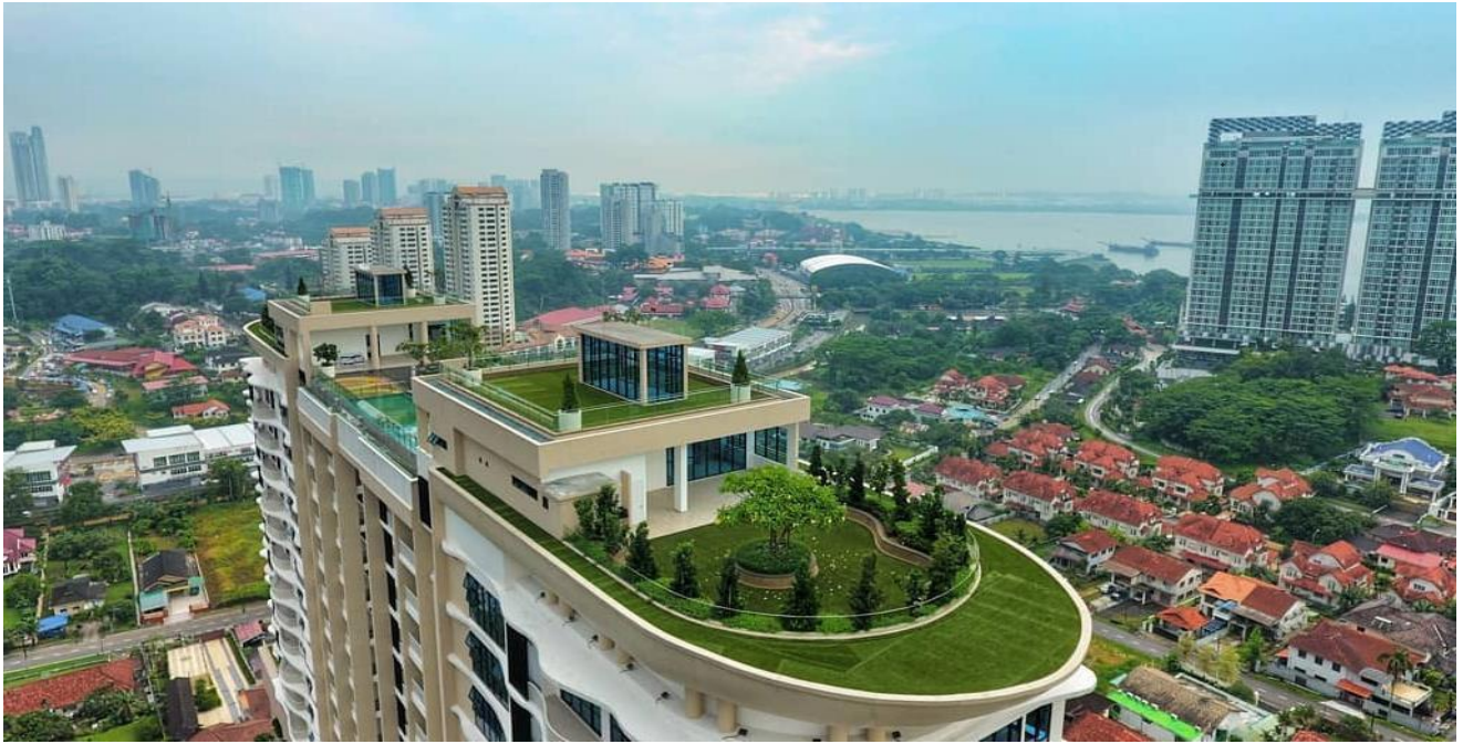
Figure 1: Green roof view of case study
