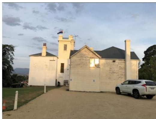
Figure 4. car park area
