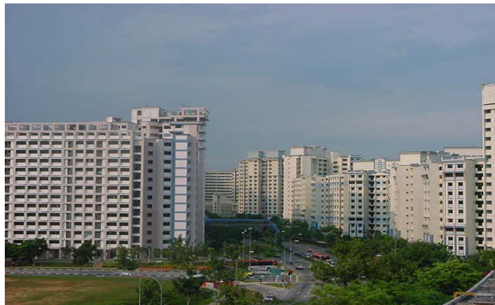
Figure 4: Sengkang public housing estate
